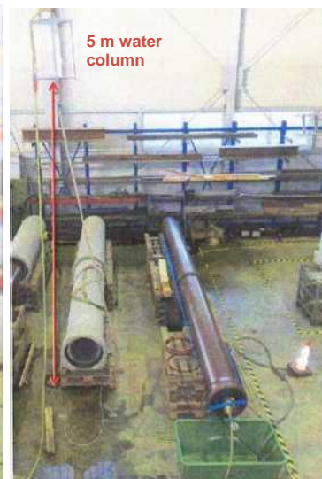
Figure 8: Leak testing, test segment 3: PVC-PVC, DN 400
