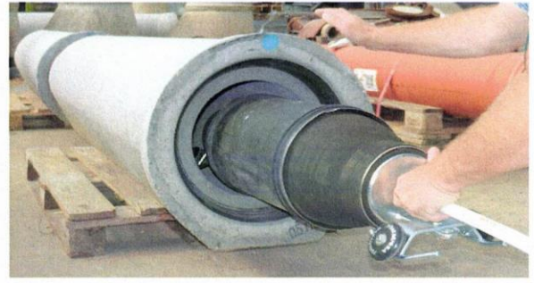
Figure 6: The Circum-MINI collar, fixed on the packer, can be positioned in the pipe.
