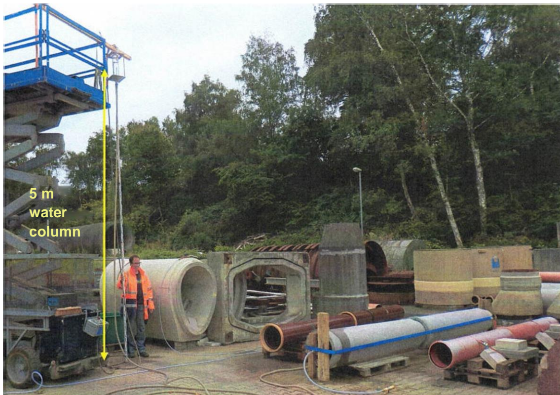
Figure 9: Test setup for the leakage test at 0.5 bar (5 m water column)
